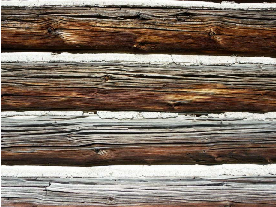
Figure 3. Degradation by UV Radiation on Cabin 1379 at the Bar BC Dude Ranch, Bar BC Condition Assessment and Report conducted by the Architectural Conservation Laboratory of the University of Pennsylvania.
