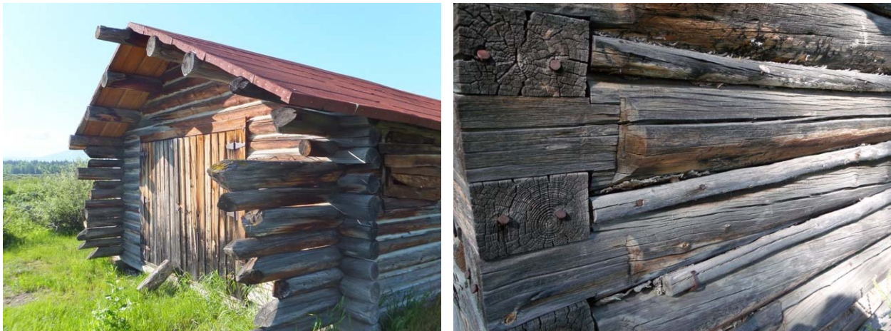
Figure 2. Cabin 1368 (left) and 1369 (right) on the Bar BC Dude Ranch, Bar BC Condition Assessment and Report conducted by the Architectural Conservation Laboratory of the University of Pennsylvania.
