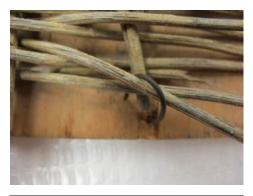
**Figure 5:** Example of wire used to attach the ends of the wicker to the plywood board.
