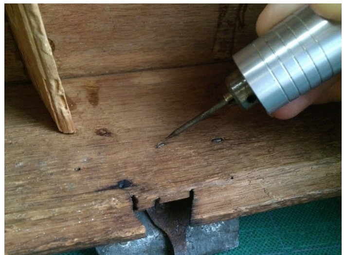
Fig 43. The tips of the nails bent on the interior were cut off using an electric rotary tool.
