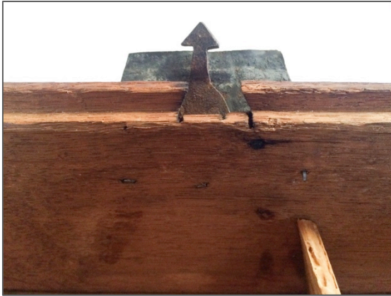
Fig. 6. The unfinished quality of the wood and misalignment of some of the case's components suggest a somewhat hasty construction.
