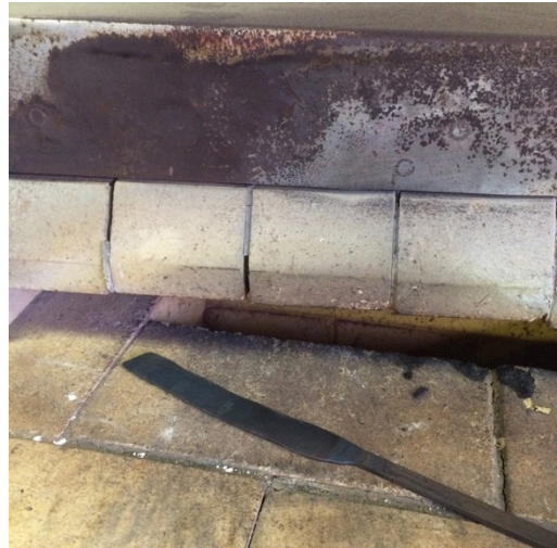
Fig 48. Piece of mild steel forged and shaped before being cut and rusticated for the replacement hinge pieces.
