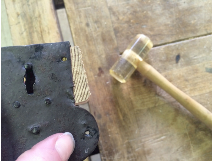
Fig 44. Distortions were corrected by hammering the metal between pieces of wood (on the left) and by using a number of other wooden tools with rounded tips (on the right)
