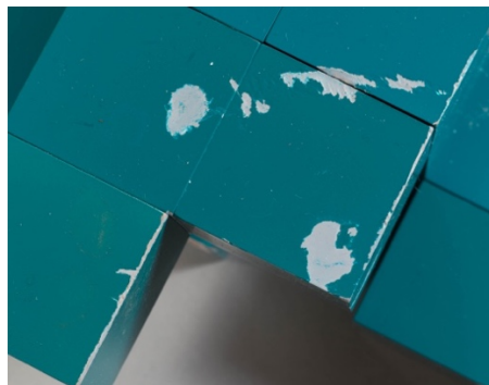
Figure 4. BT condition: abrasions
