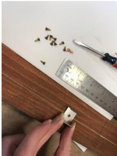
Figure 5. Toned beam with markings in chalk, a metal clip in position, ¼ inch screws, and a flat head screwdriver. (Image courtesy of Dr. Stoner.)
