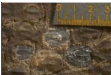
Fig.15 detail of spalling, ( \frac{1}{10}^{\text{th}} mm), before treatment
