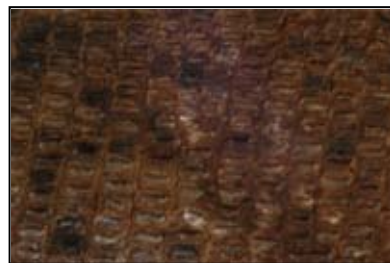
Fig.16 detail of spalling 6x magnification, before treatment
