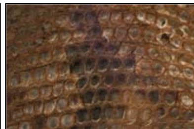
Fig.17 detail of cracks, before treatment
