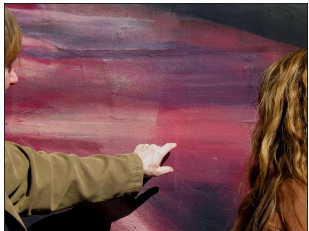
Fig 5 – Detail of Richard Wolbers pointing out chalking and fading on paint surface to the artist, Meg Saligman. Photo of Philadelphia Muses , Meg Saligman, 1998 by Joyce Hill Stoner, 2005
