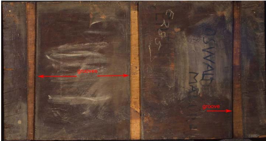
Figure 7: Verso of panel showing vertical grooves
