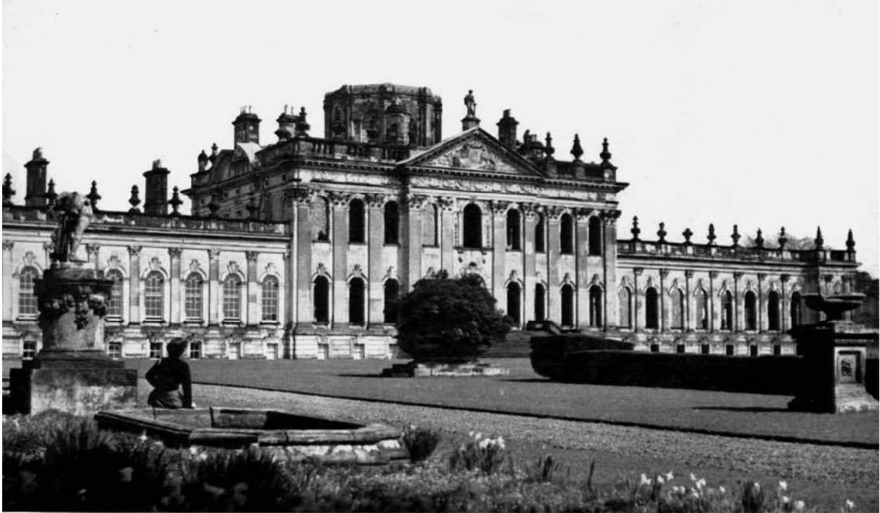
Figure 1-2. Castle Howard, south front after fire of 1940.
