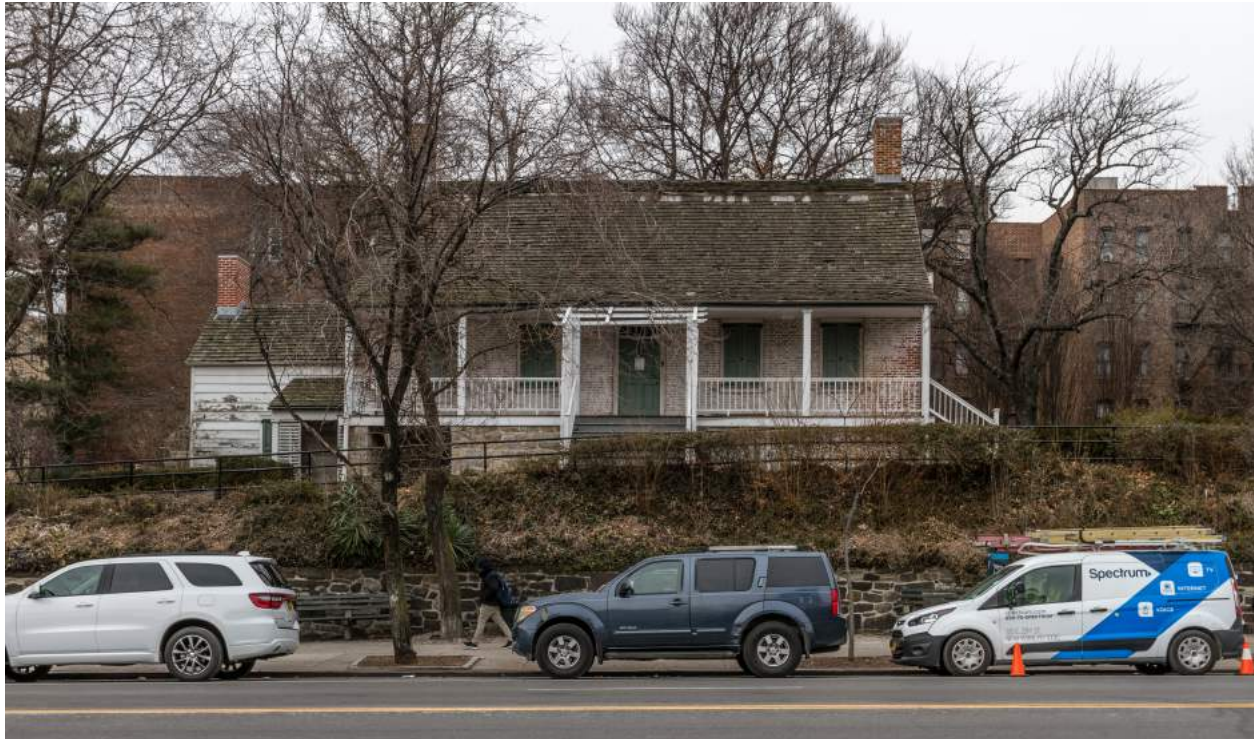
Figure 4-11. Dyckman Farmhouse (south elevation)
