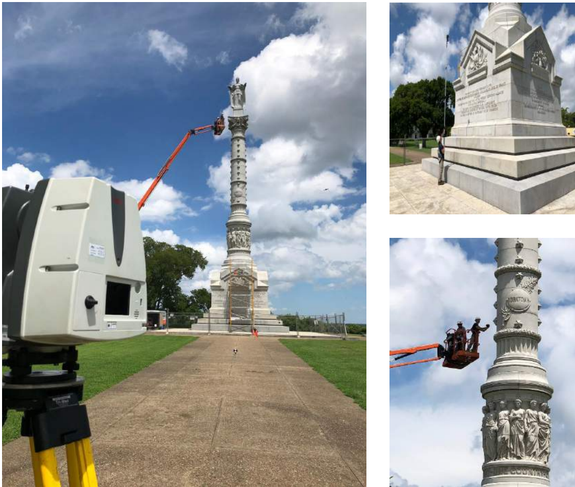
Figure 3-23. HABS crew using hybrid recording method of Yorktown Victory Monument, in Virginia.
