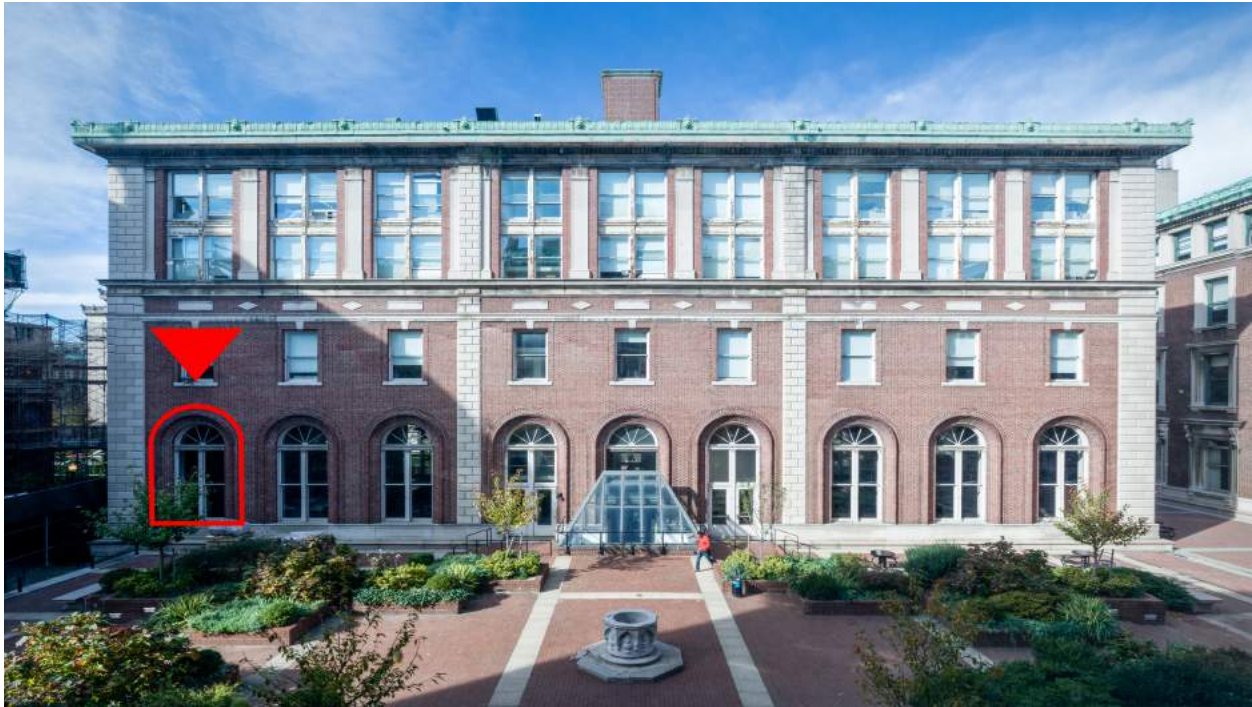
Figure 4-8. The red arrow highlights the window studied in this experiment, located on the east elevation of Avery Hall.
