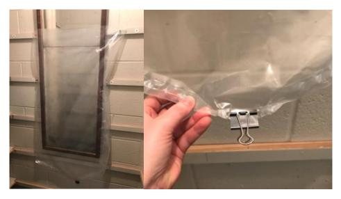
Figs. 6,7. The polyethylene bag created to contain the mercury drips on mirror.
