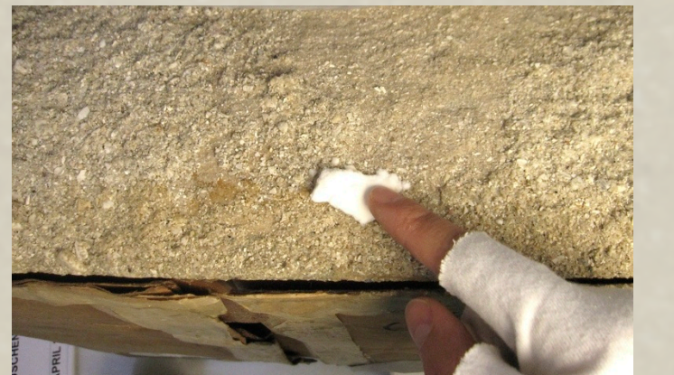
Figure 7: Stain removal (DT)
