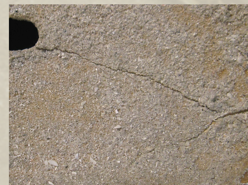
Figure 11: Detail Crack (BT)
