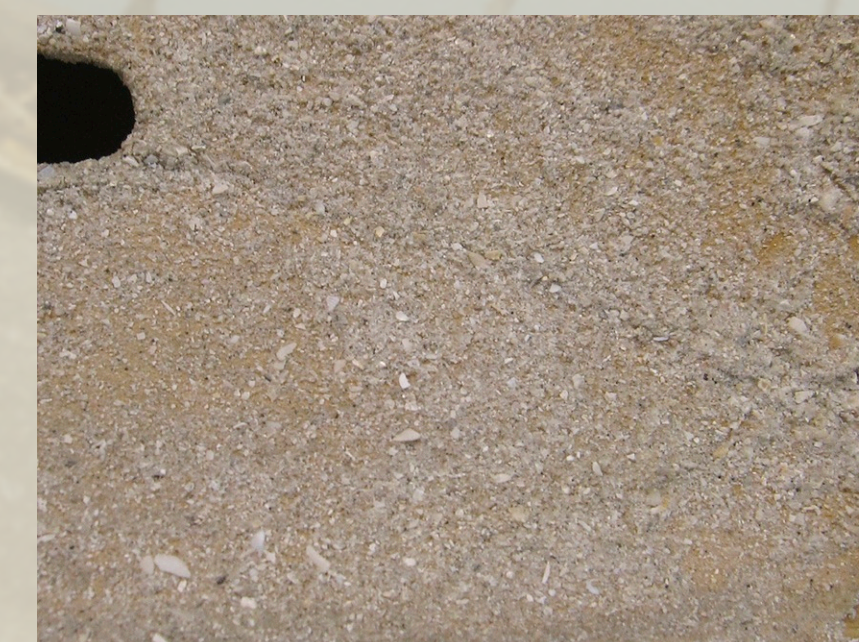
Figure 12: Detail Crack (AT)
