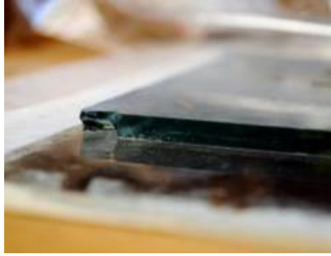
Fig. 8 Detail of chipped glass.
