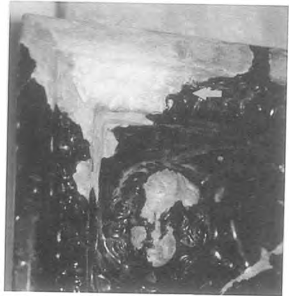
Figure 5b. Detail of applied putty, burnished but uncoated.
