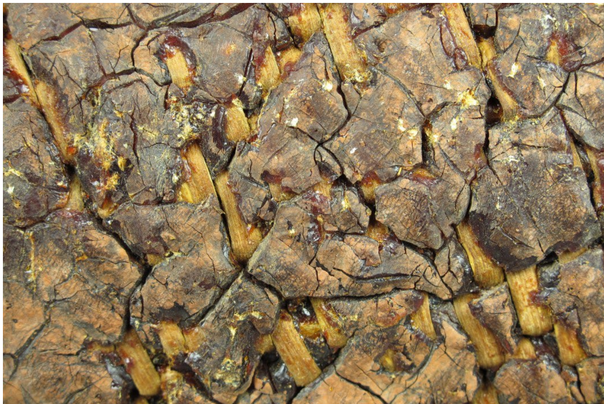
Fig. 6. Darker, opaque pitch exhibiting deep cracking, discoloration, and loss (Courtesy of Marilen Pool)
