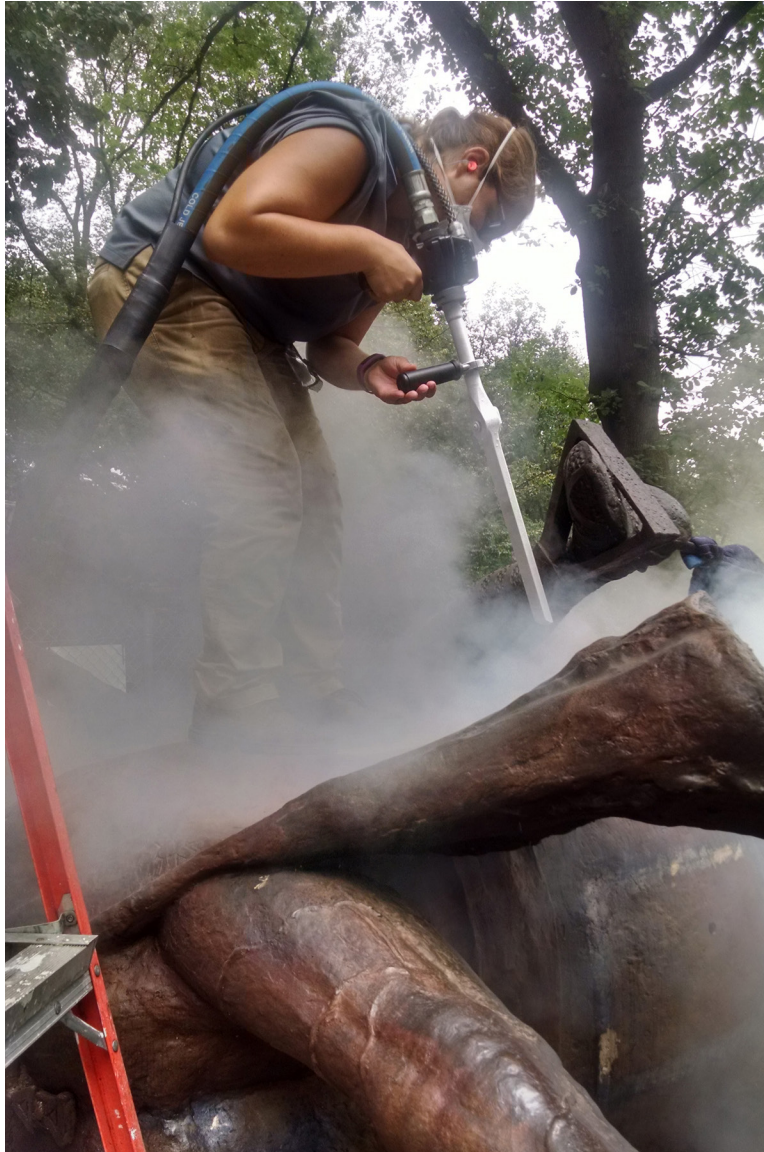
Fig. 10. Dry ice blasting while sculpture was deposed from base
