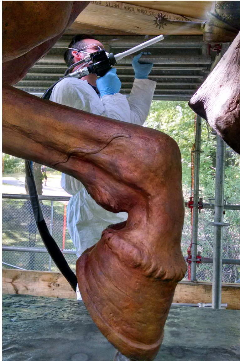
Fig. 13. Blasting with short conical nozzle in the more restricted workspace of the scaffolded monument
