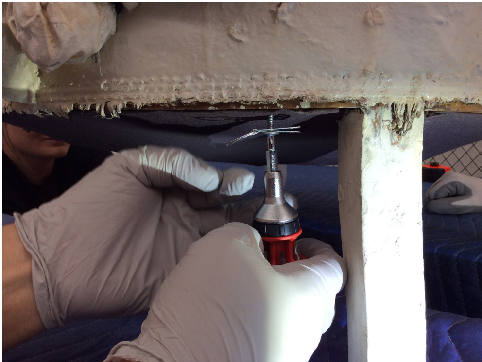
Fig. 13. One of three D-rings being installed to the wooden framework. The D-ring is used in transit and flipped up for exhibition.
