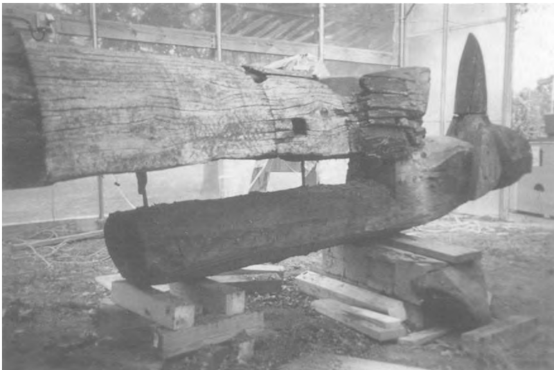
Figure 3. Eagle figure being lowered away from the pole to gain access to cracks and rot.
