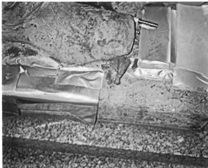
Figure 9. Self-base of Christopher Columbus masked off for the cleaning tests, 1992.
