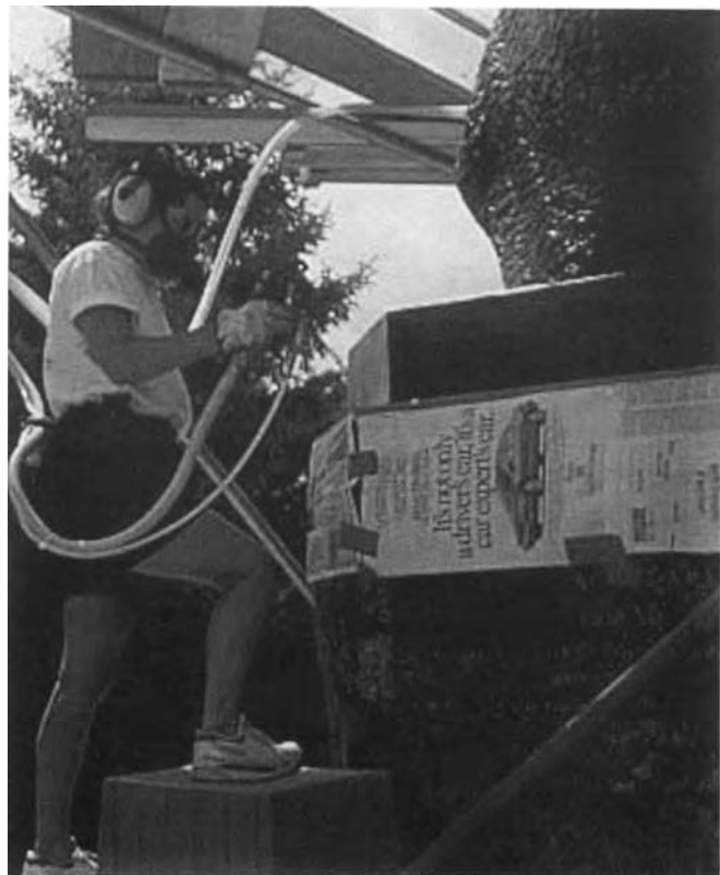
Figure 13. CTA staff applying Incralac lacquer to the self base of Leif Erickson , 1996.
