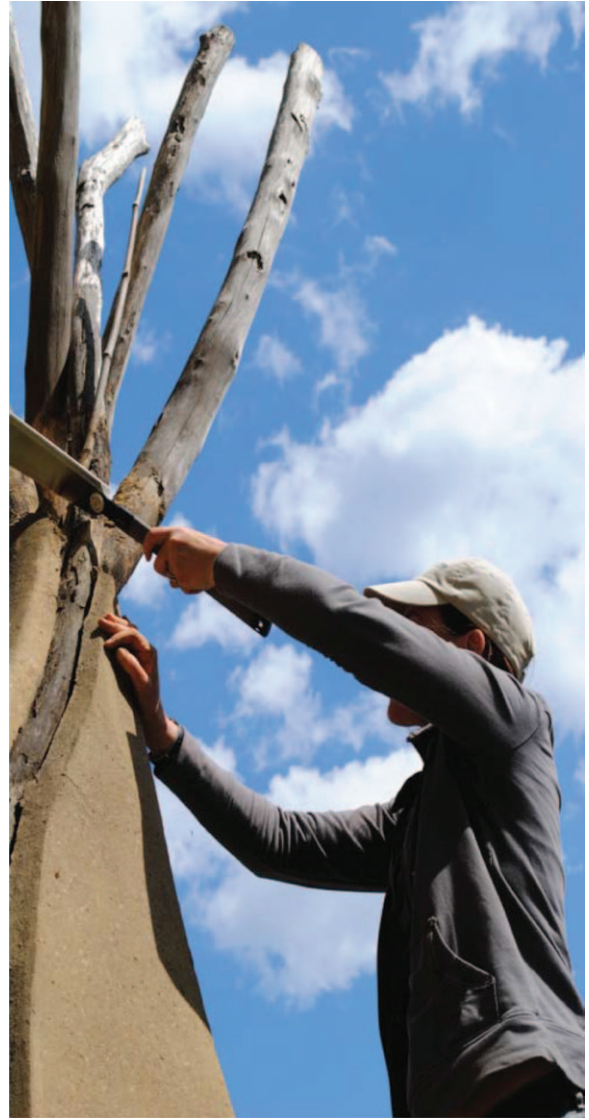
Fig. 10b. Conservator Kelly McHugh uses a Japanese saw to remove a piece of bamboo (Courtesy of G. Joice).
