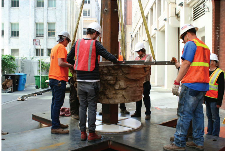
Fig. 13. Assembly of sections onto new mount, lifting the sections from steel beams that were temporarily attached (Courtesy of Ursula von Rydingsvard, photograph by Emily Hamilton)
