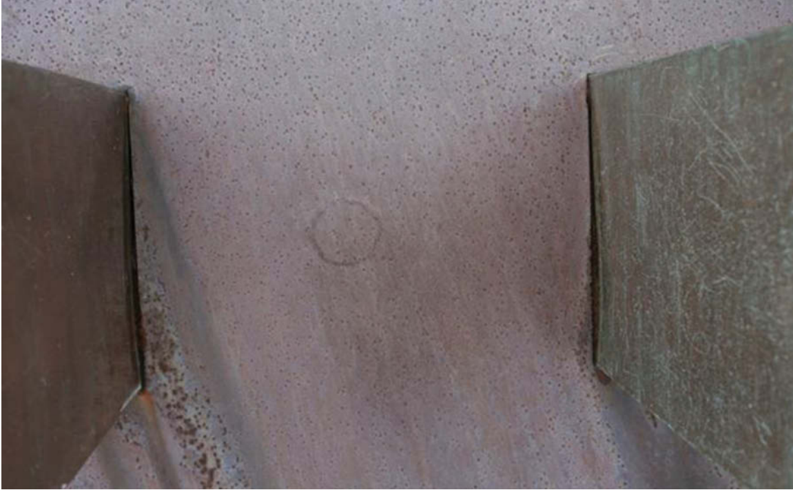
Fig. 15. Inward bowing of the bronze prongs on the Oberlin Plug due to expansion of iron corrosion products in the gap between the bronze and the COR-TEN steel (Courtesy of John T. Seyfried, ICA)
