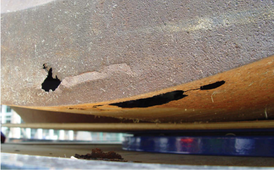
Fig. 10. Severe corrosion at interface between side chamber body and face of the Saint Louis Plug, due to humid micro-environment in the space created by the internal angle iron (Courtesy of Russell-Martí Conservation Services, Inc.)
