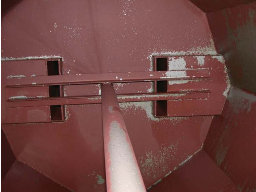
Fig. 5. View inside the large central chamber of the Saint Louis Plug, showing the central shaft running horizontally through the body (Courtesy of Russell-Marti Conservation Services, Inc.)
