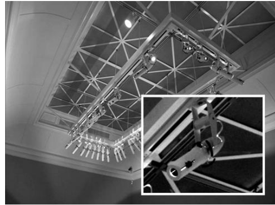
Figure 3. Superstructure holding the projector lamps. Inset of an LSI lamp projector lamp unit.
