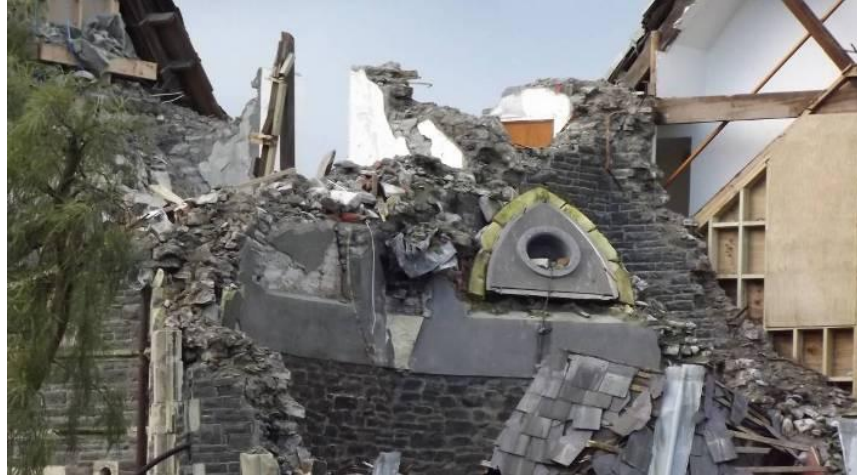
Fig. 3 Damage after February 22, 2011.
