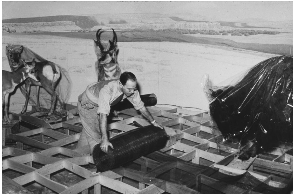
Fig. 3. Foreground artist George Frederick Mason laying down wire mesh over wood contours to create the ground terrain in the American bison/pronghorn antelope diorama (1942) (Courtesy of the American Museum of Natural History)
